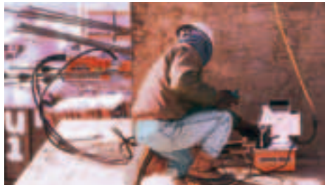
The PE60 used for pre-stressing.
