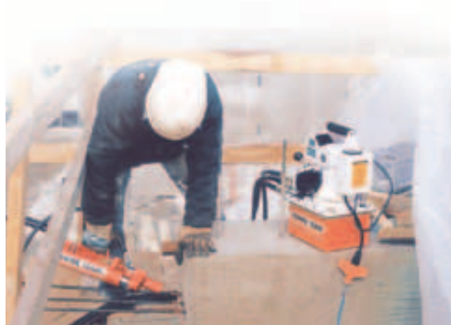
The PE60 used for pre-stressing.
